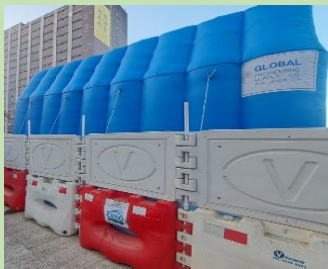
設置可重用的隔音充氣屏障 Installation of Reusable Inflatable Noise Barriers
